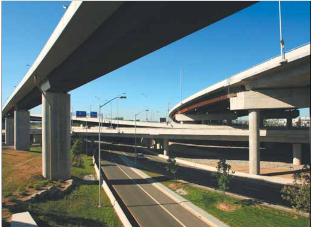
Bridges for outbound traffic to Hwy 409 at Pearson Airport, Toronto. Bridges built by Bot Construction.
